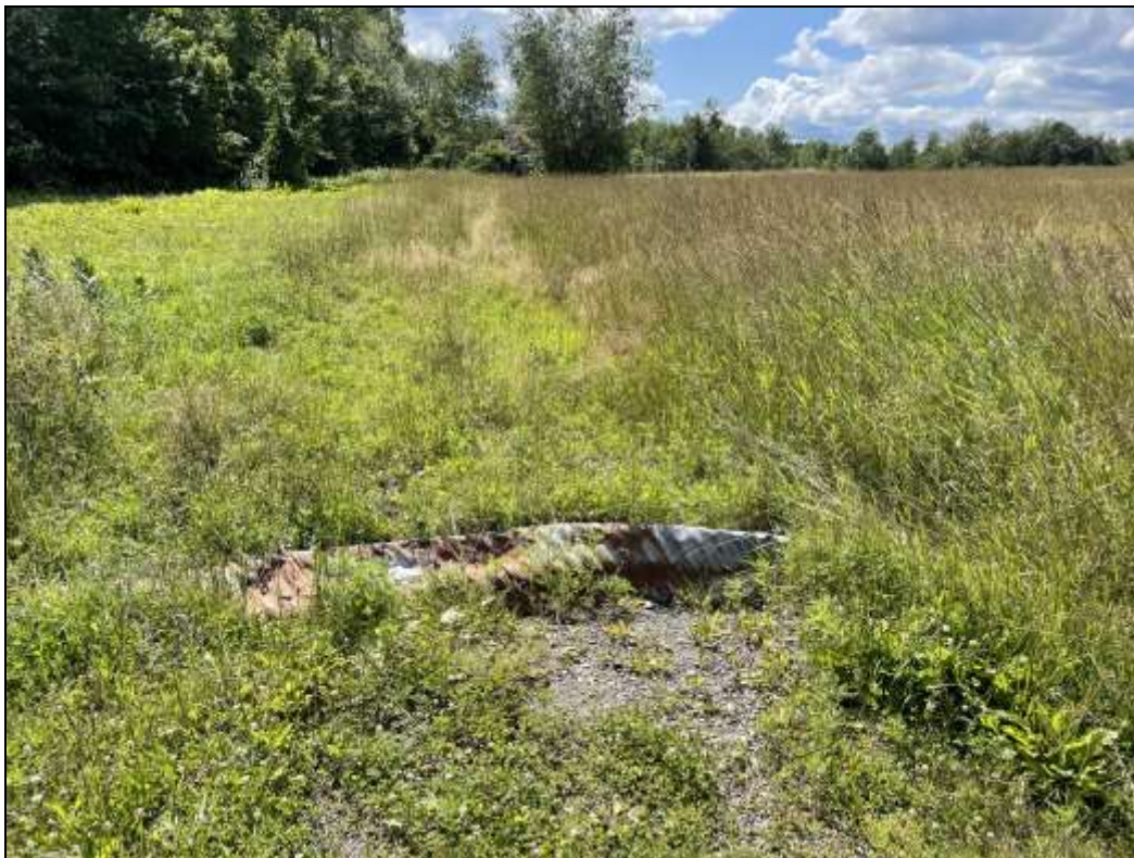
Damaged culvert at the head of Wetland 2 near southeastern corner of Southern Field
