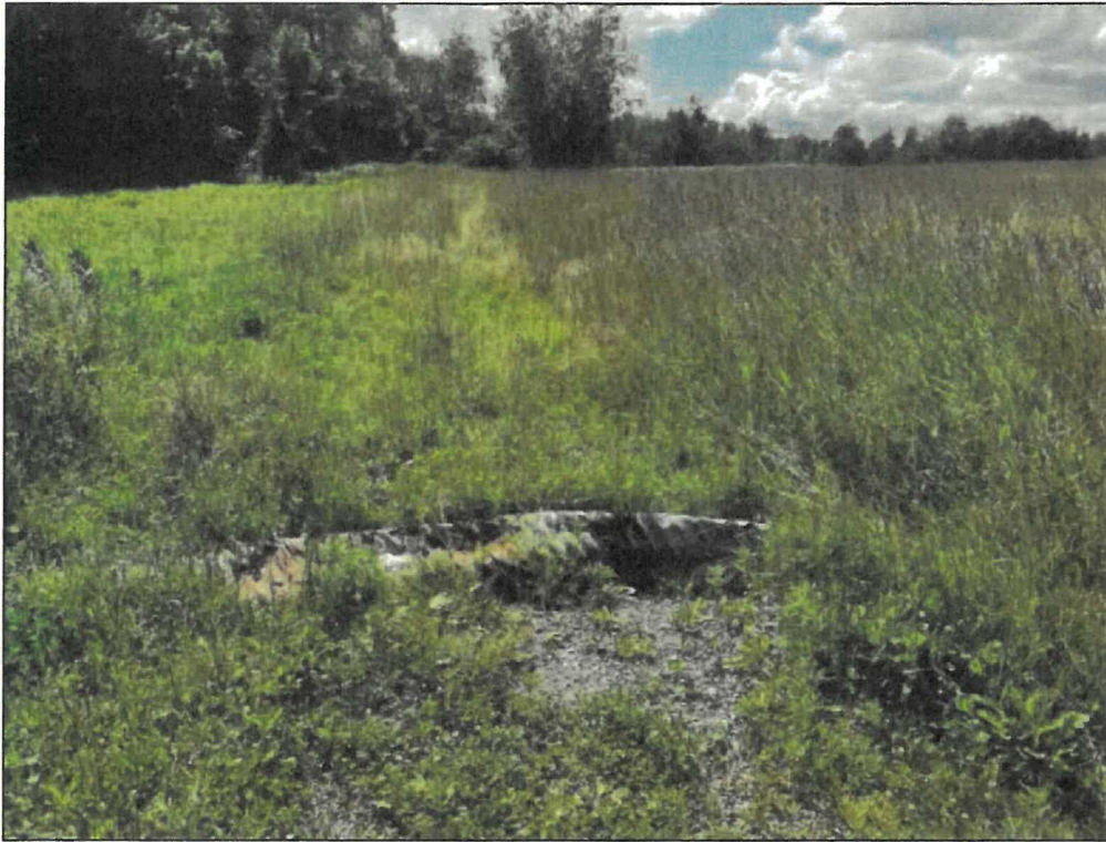
Damaged culvert at the head of Wetland 2 near southeastern corner of Southern Field
