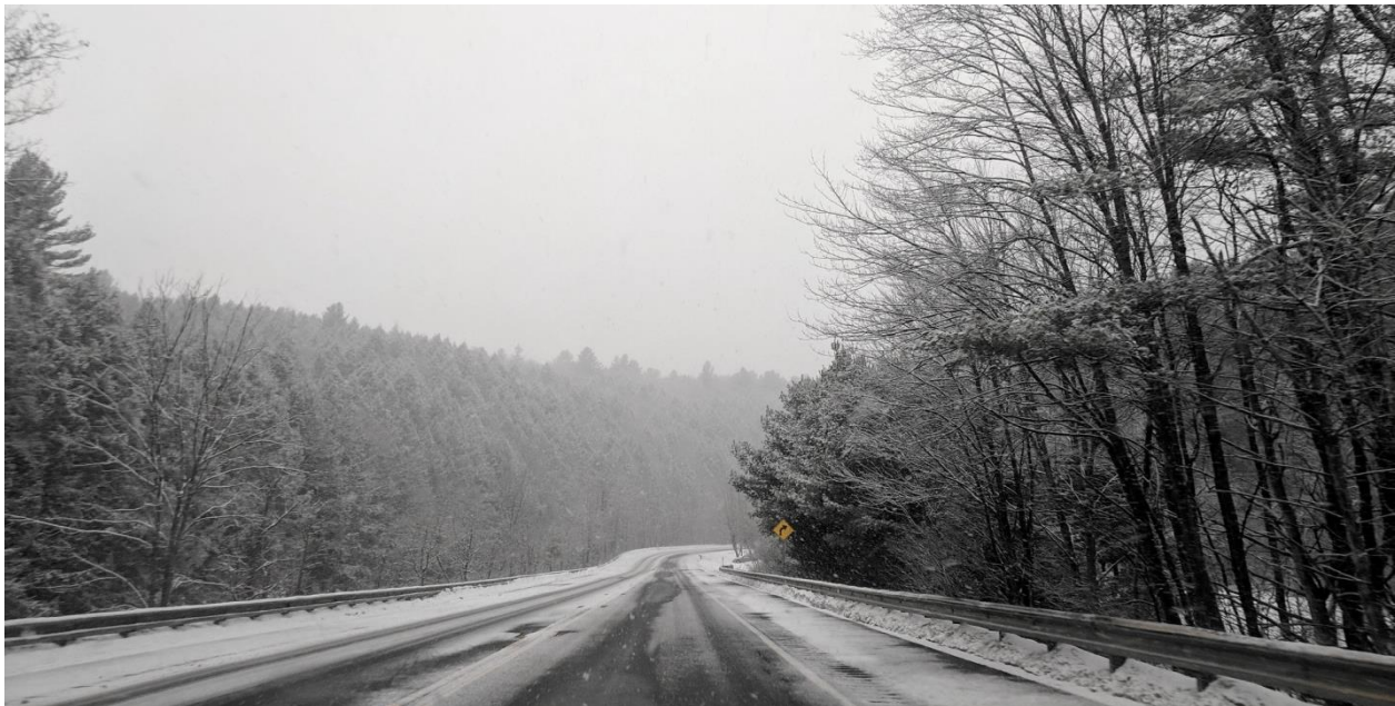
MA Route 9, the major east-west route in the area, is a hilly and winding road which can be vulnerable to winter hazards and downed tree limbs. Credit: Wikimedia Commons users John Phelan (top) and JJBer (bottom)
